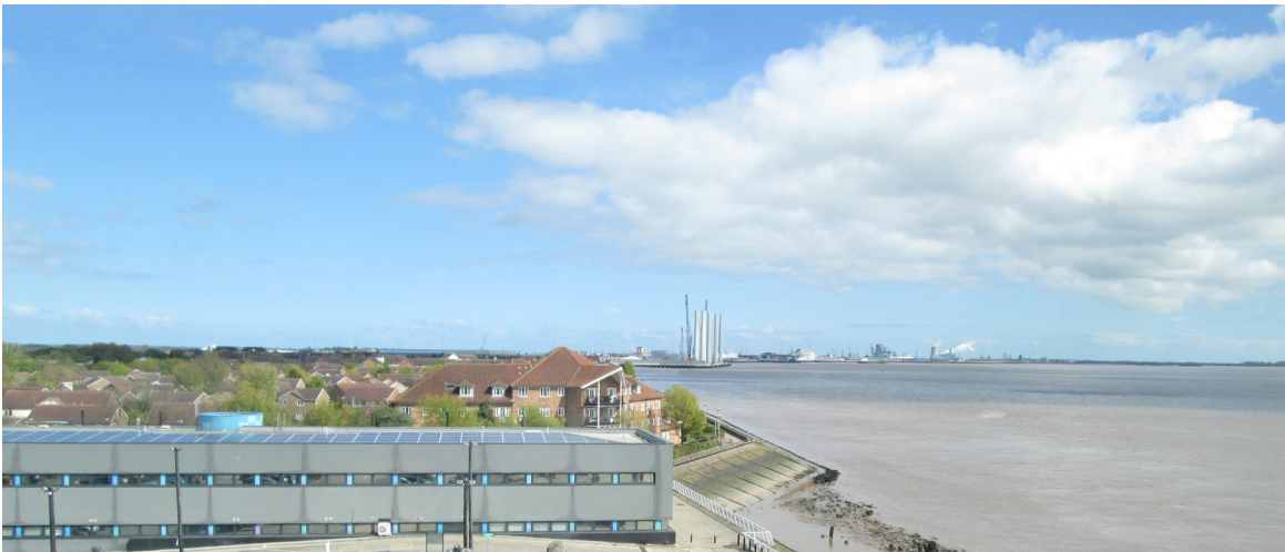
Fig. 5.3 Siemens' wind turbine manufacturing facility seen from the Deep (source: Enrico Tommarchi, 2017).
