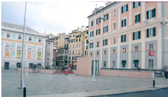
Fig. 2.10 Piazza Caricamento being repaved (above) and finished (below) (source: Arkos Dossier 2004).
