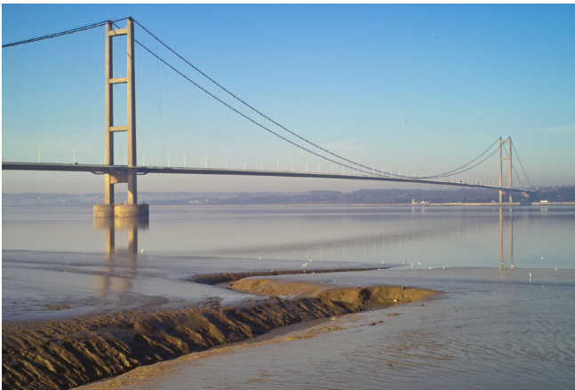
Fig. 5.6 Humber Bridge. (source: D. Wright [CC BY 2.0 - https://creativecommons.org/licenses/by/2.0 ]).
